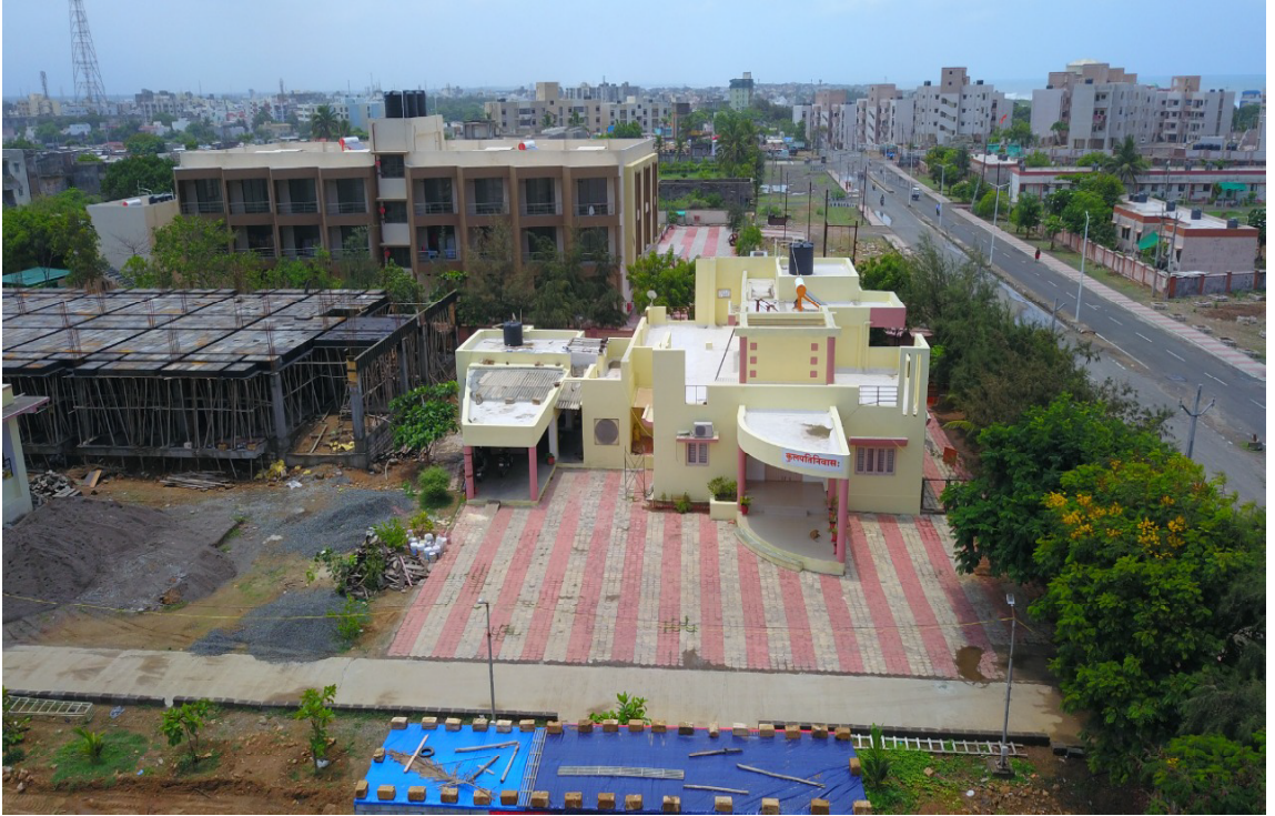
VICE-CHANCELLOR'S BUNGLOW & GUEST HOUSE UNDER CONSTRUCTION
